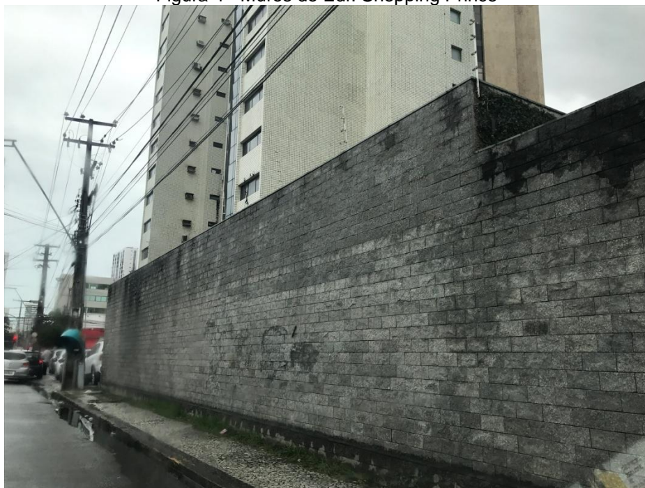
Figura 4 - Muros do Edf. Shopping Prince
